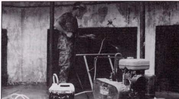
A new wet sandblaster from Kennards Hire was used by the Army to restore gun fortifications at North Head in Sydney
