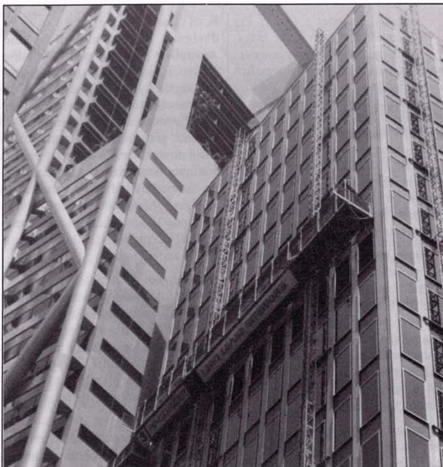
Hi-Climber in use on the refurbishing of No 1 Castlereagh Street, Sydney
